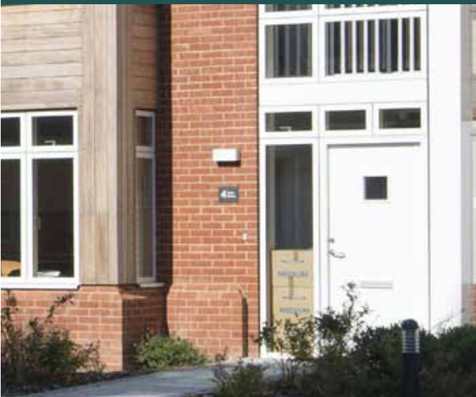
INWARD OPENING GROOVED FLUSH ENTRANCE DOOR AND VELFAC 200 FIXED SIDE/TOP LIGHT
