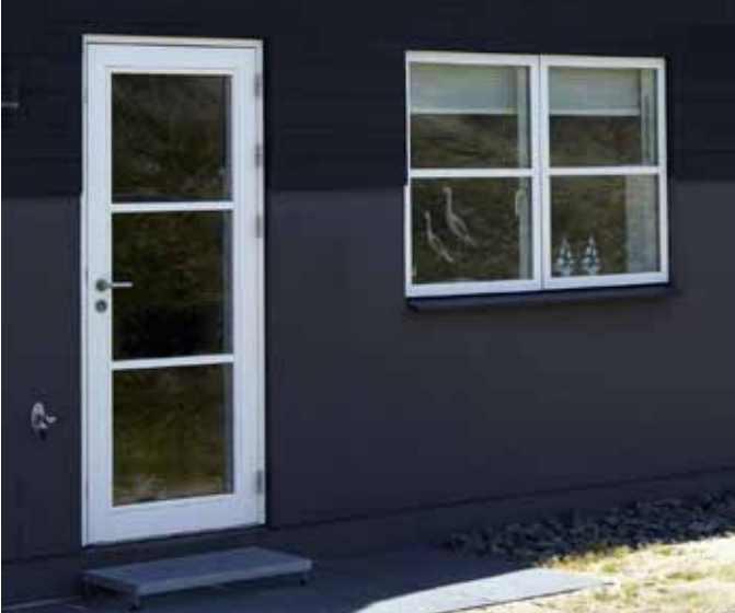
OUTWARD OPENING GLAZED ENTRANCE DOOR WITH GLAZING BARS AND A VELFAC 200 WINDOW
