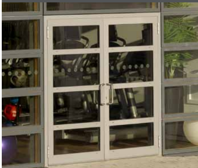
2-LEAF DOOR WITH CRANKED PULL HANDLE AND GLAZING BARS IN A VELFAC 200 WINDOW FAÇADE
