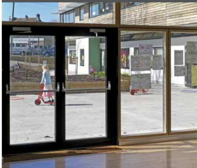
2-LEAF ESCAPE DOOR WITH PANIC BAR AND DOOR CLOSER IN A VELFAC 200 WINDOW FAÇADE
